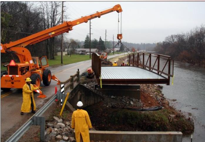
**Installation:** Virtually all of our bridges can be installed in one day. Larger bridges that have to be spliced for shipment can be easily bolted together (no field welding required) and erected in hours instead of days as required by "stick-built" bridges. This allows for minimum disruption of the job site and gets people walking or driving across your bridge as quickly as possible.
