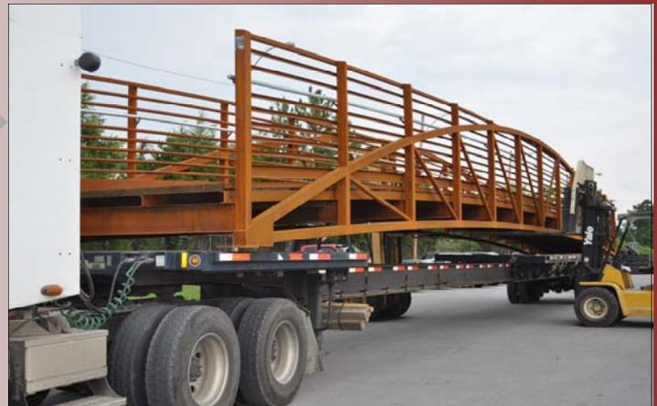
*Loading of a Crossbow Style bridge with two forklifts ►*
